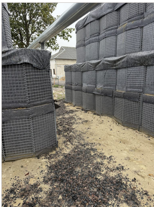
Filled HDGDEF units with geotextile lining
